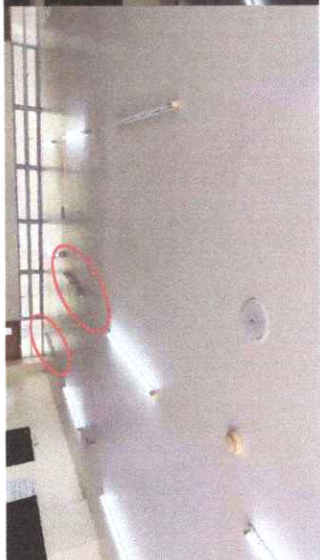
EXISTING BUSTED LIGHTS NOTE: REPLACE ALL BUSTED LIGHTS AND REPAIR WIRINGS
