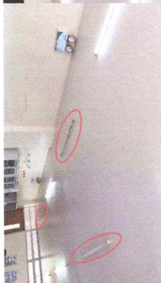
EXISTING BUSTED LIGHTS NOTE: REPLACE ALL BUSTED LIGHTS AND REPAIR WIRINGS
